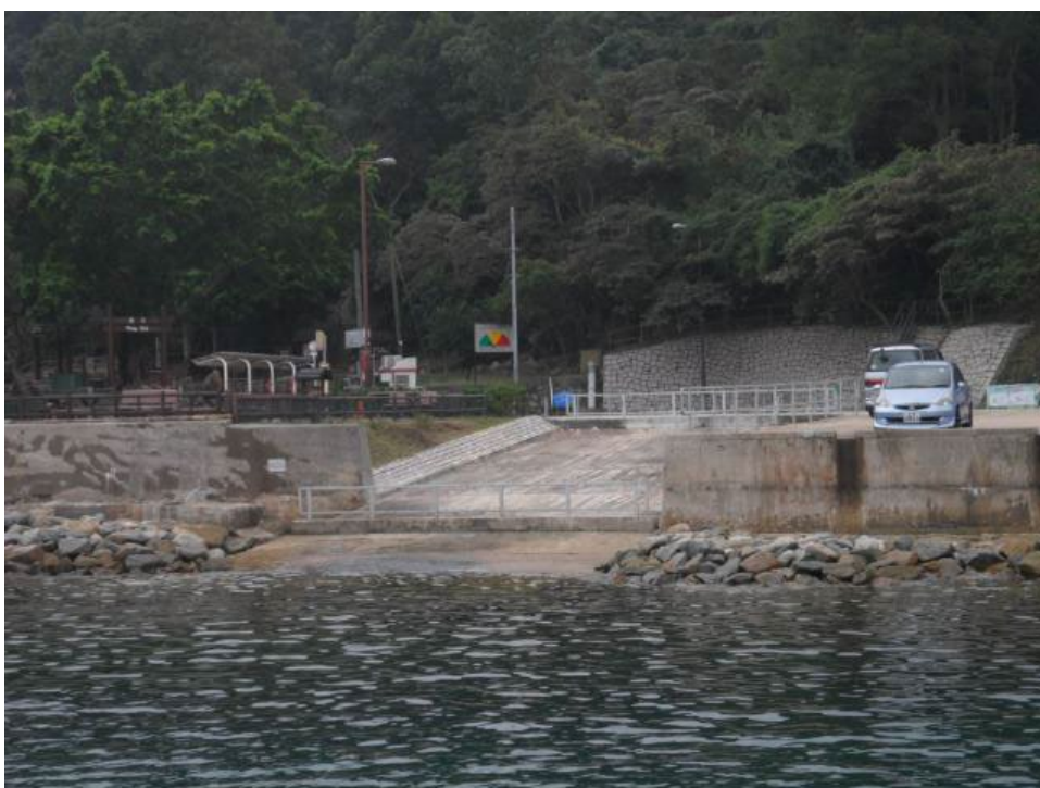
Example: Wong Shek Slipway
