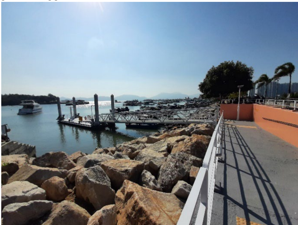
Example: Floating pontoon at Tuen Mun Area 27
